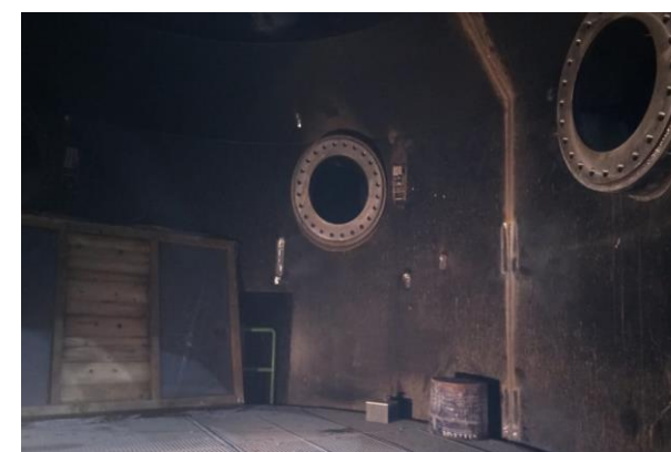
UNIT-1& 2, TURBINE HOUSING & DISTRIBUTOR COMPLETED
