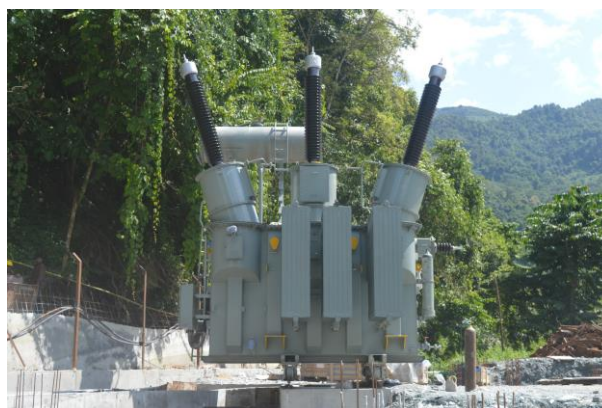
10MVA STATION TRANSFORMER ERECTION COMPLETED
