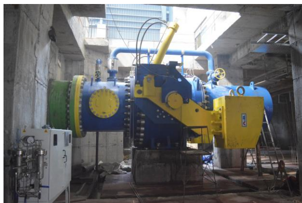
UNIT- 2 MIV ERECTION COMPLETED
